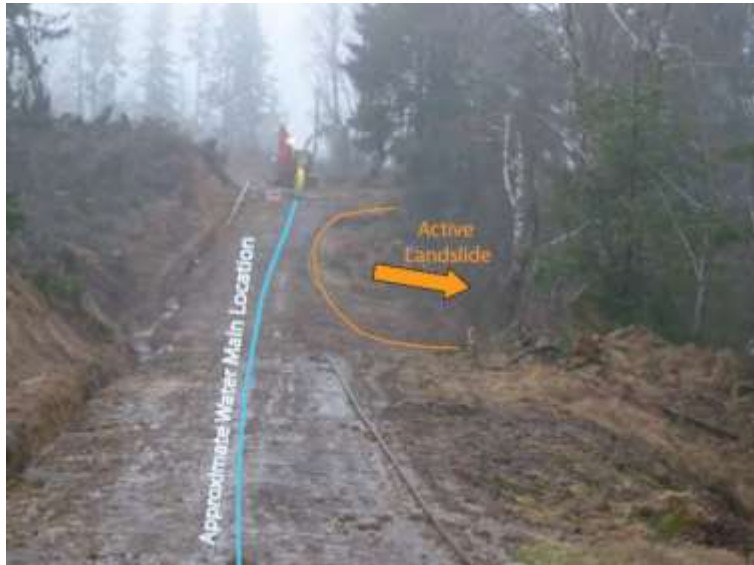
Figure II-59. City of Astoria's potable water main threatened by an active landslide.
